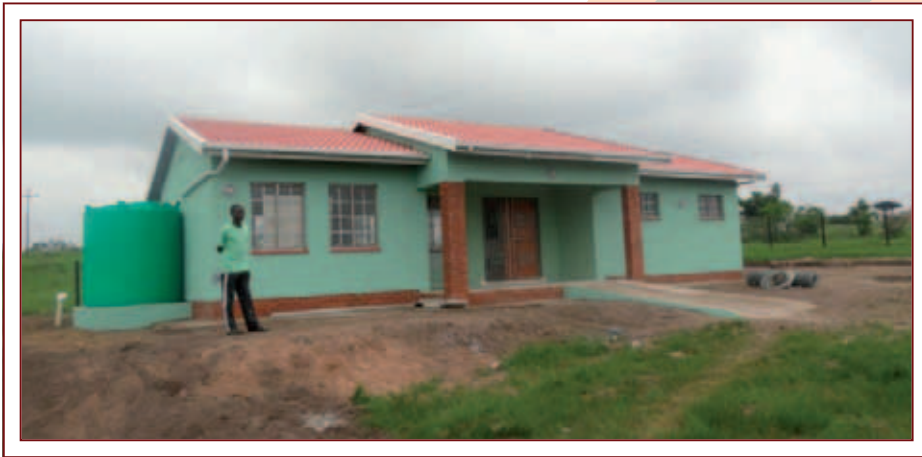
Newly Built Project at St. Nivard's Centre – Umzinto
