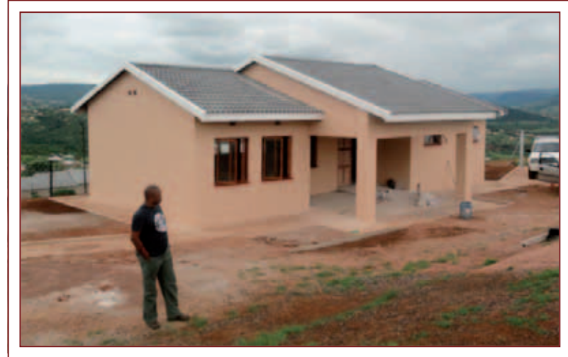
Newly Built Project at Umsunduzi Resource Centre – KwaXimba
