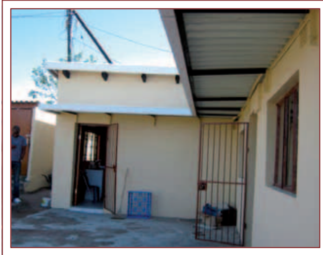
Repairs & Renovation – Folweni Community Centre
